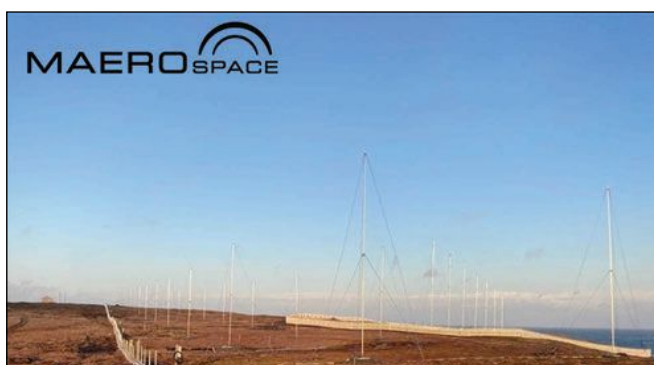
▲ Fig. 4 Maerospac HFSWR installation, Cape Race, Newfoundland. Source: Maerospac Corporation.
